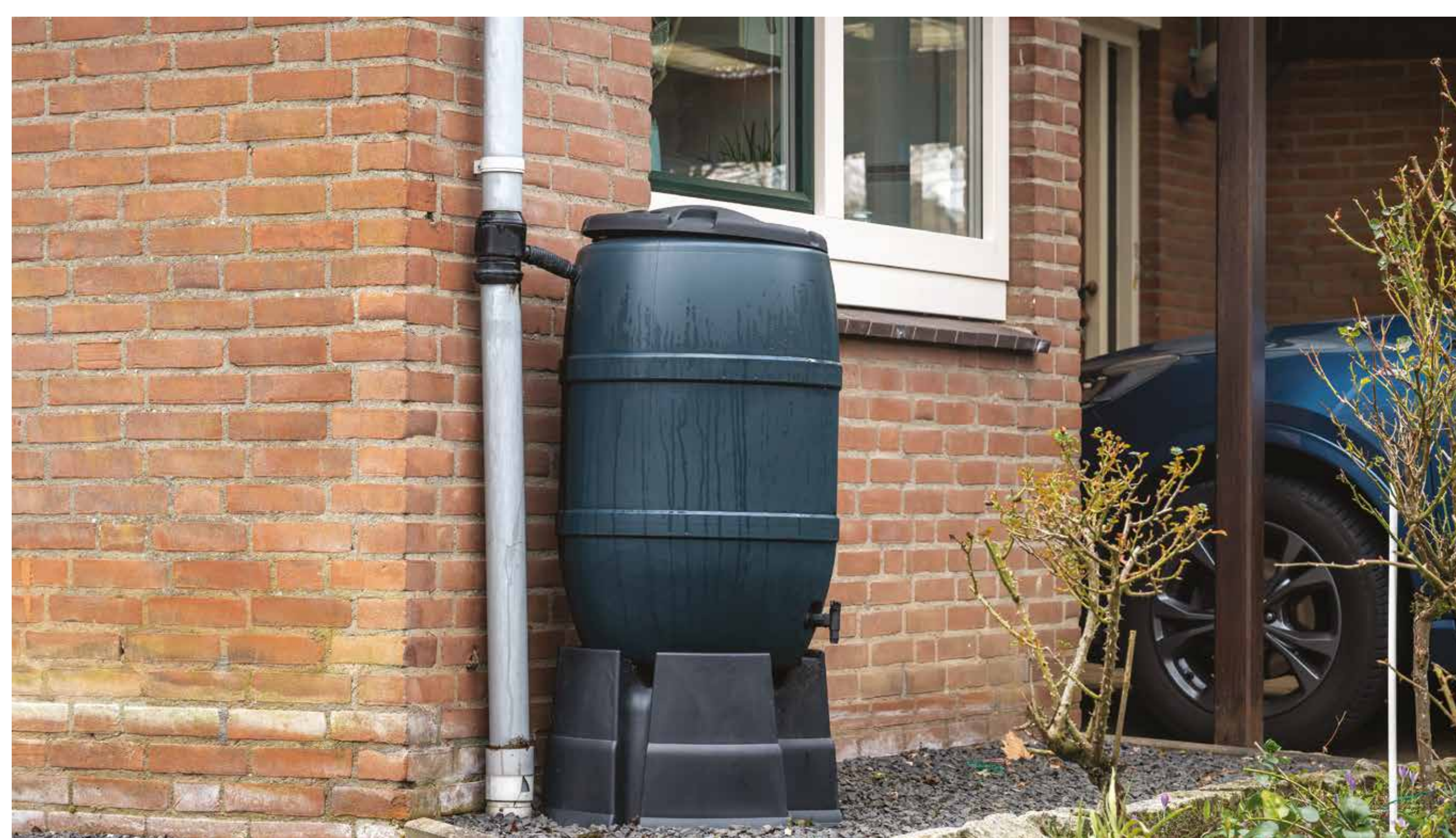
Water butts one of the most common measures for property-level SUDs, collecting rainwater.
