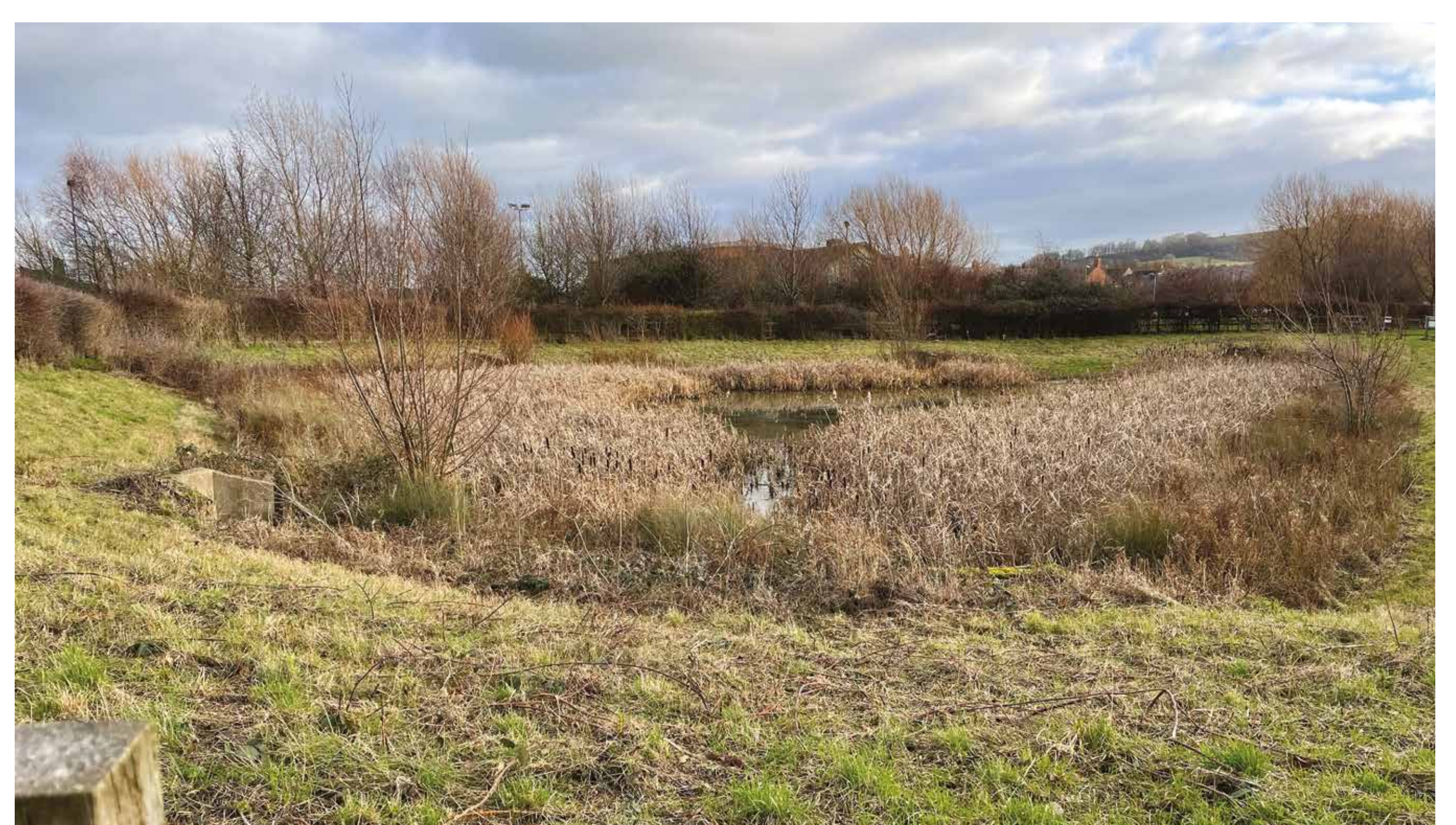
Detention basins providing attenuation during heavy rainfall, but functions as a recreational facility during the dry periods.
